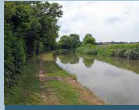
Figure 66: The Canal between Stowehill and Nether Heyford
