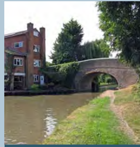
Figure 58: Bridge No 27 at Flore Lane Wharf
