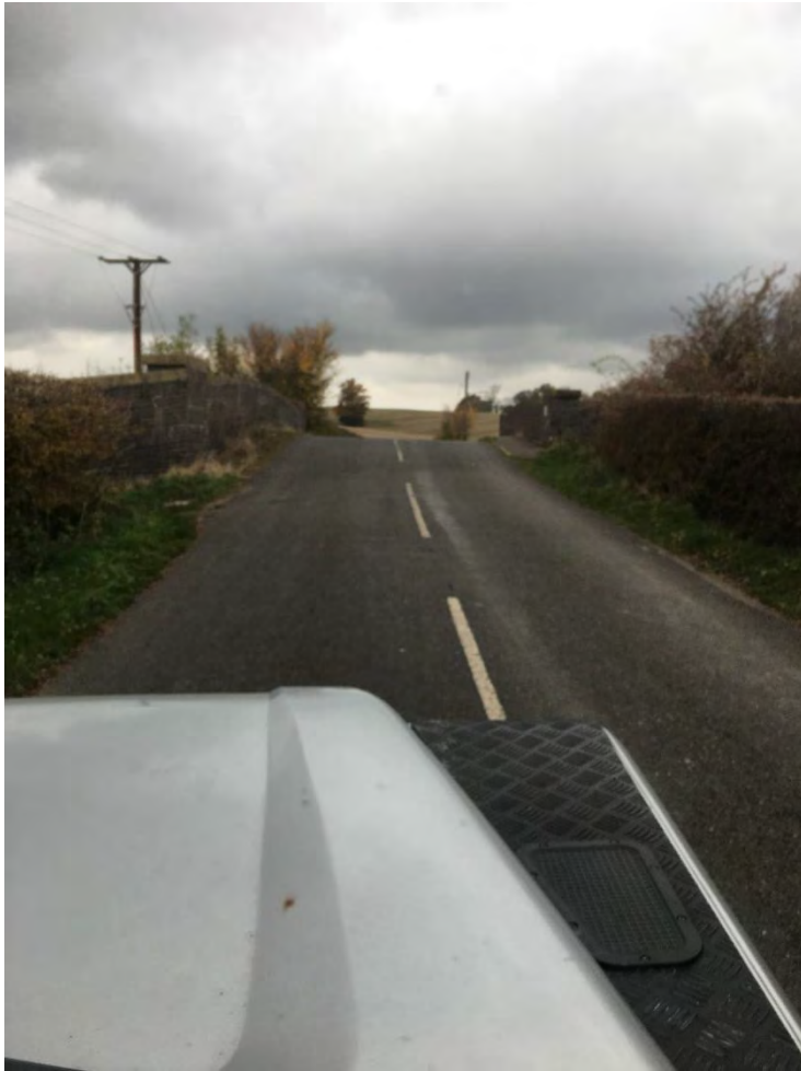
Vehicle access over bridge on Station Road
