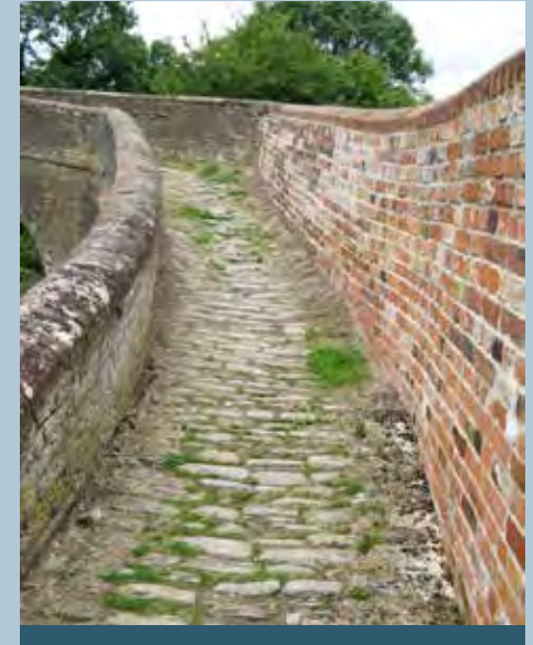
Figure 69: Detail of the Turnover Bridge (Bridge No 47)
